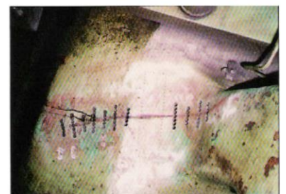
DRILLING FOR BOTH METALOCK AND MASTERLOCK
