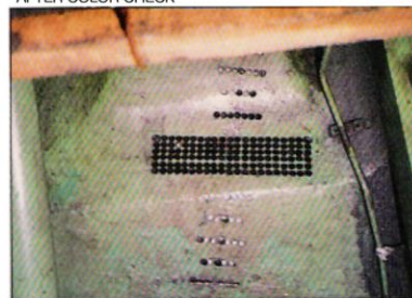
SLOTING FOR ERILLED AREA
